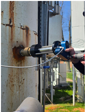
Figure 16. Withdrawal using the remover tool.
