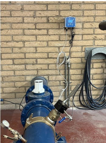
Figure 15. Field installation on a main.
